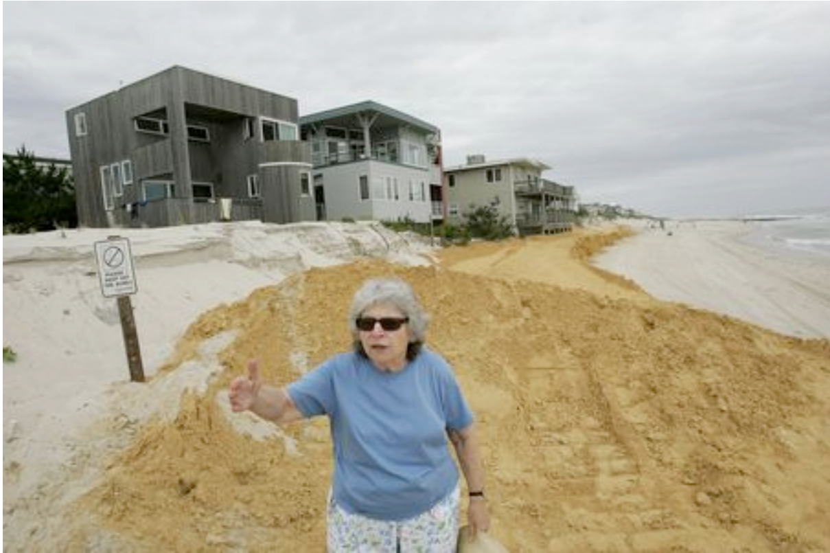
(AP Photo/Mel Evans) Arlene Pollack, 77, stands on emergency dune and beach replenishment near her home, left, and two others on the Atlantic Ocean in Harvey Cedars, N.J., Monday, July 14, 2008. The borough trucked in 3,000 cubic yards of sand on an emergency basis to protect the homes there during the first week of July -- but two-thirds of it has already washed away.
